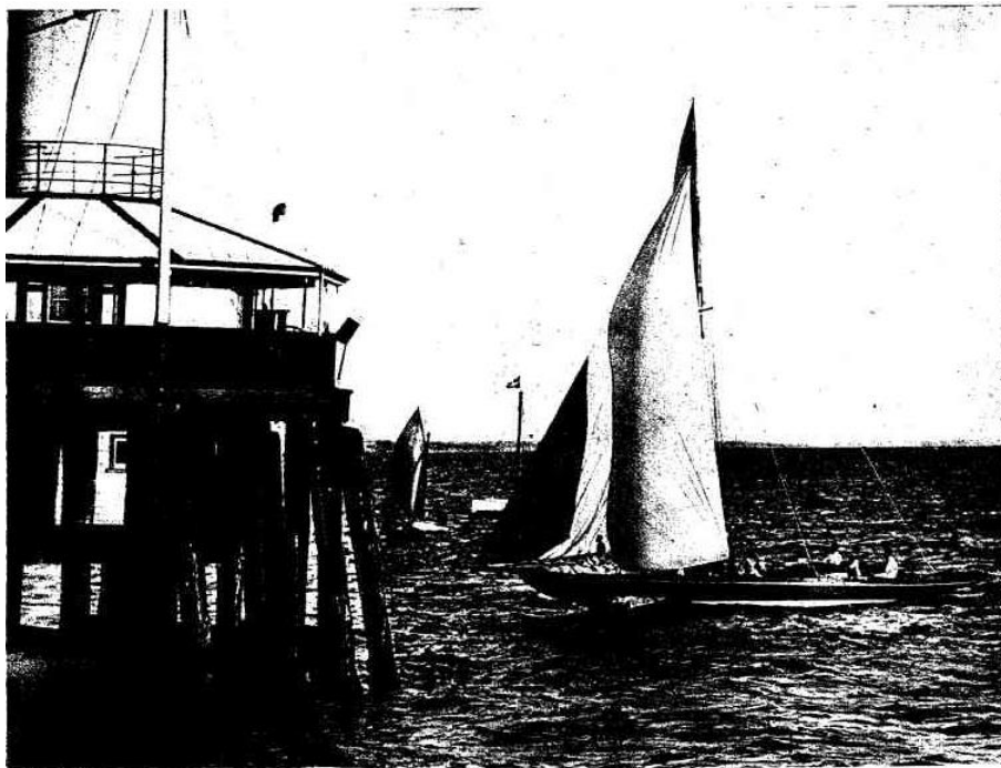
CULWALLA III. FINISHING.
